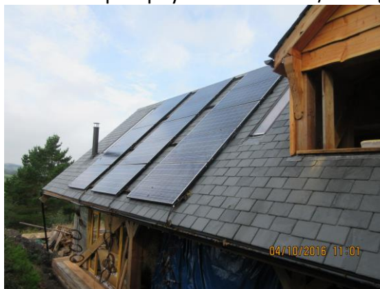
Exton, Self-build local affordable home under construction (2016)
