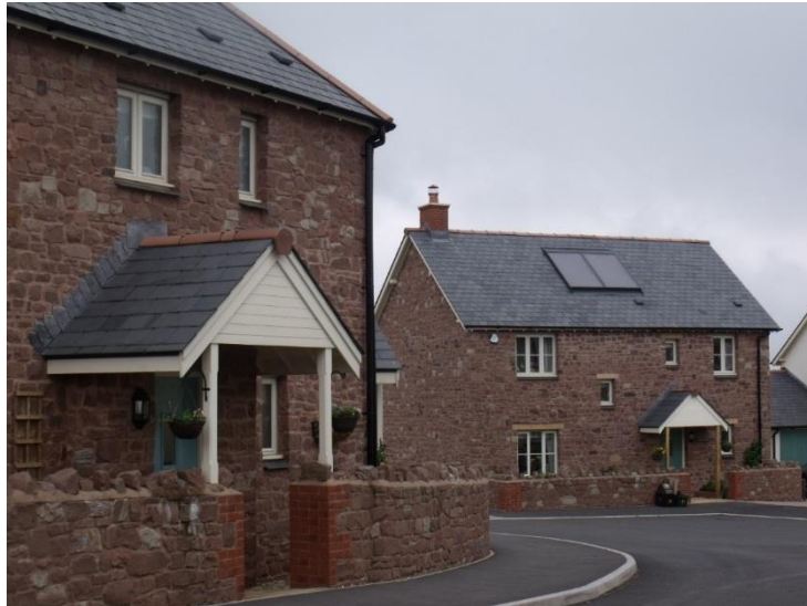
CUTCOMBE Permission granted for 25 dwellings (13 open market 12 affordable) on the former Livestock Market site
